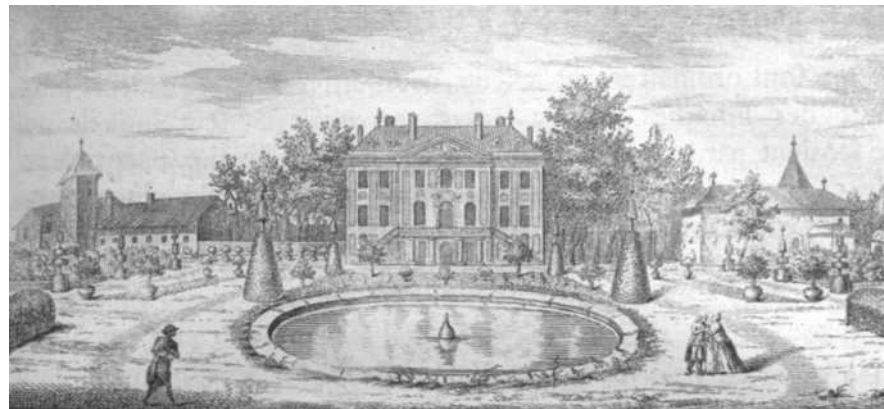
FIGURE 2.3. Bonnet's house at Genthod, with a part of the French garden in the middle and two kitchen gardens on the right and on the left, from Bonnet's Oeuvres complètes, ed. in-4°.
